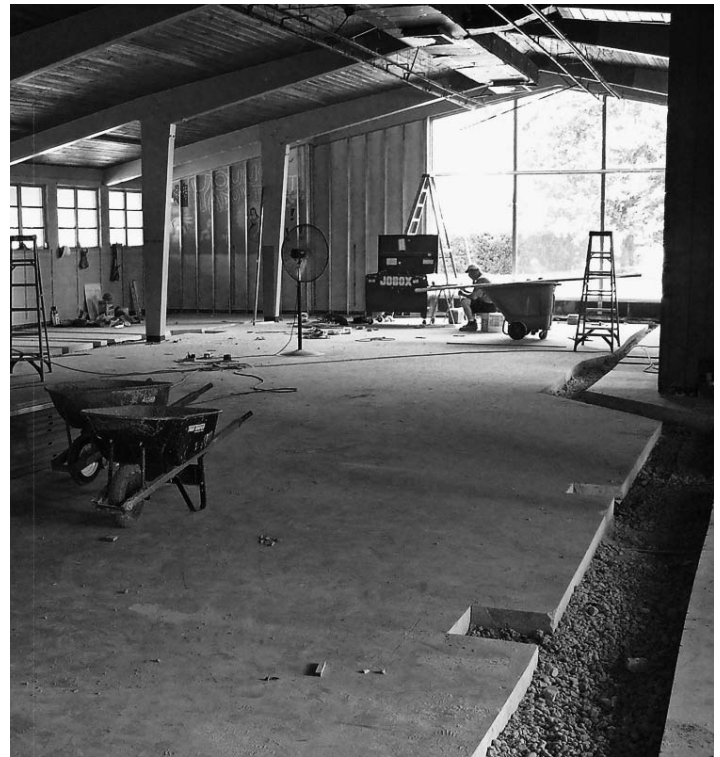
Renovations on the Westover Hills Library have begun in earnest. Channels have been cut in the concrete floor to remove existing duct-work. In the next few weeks, work will begin on the installation of an all metal roof and the extensive rewiring of the building will take place as well. The Library was originally built in 1959. Photo: Clay Dishon
